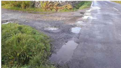
Resp5: Junction of access at Lorgba onto main A847
