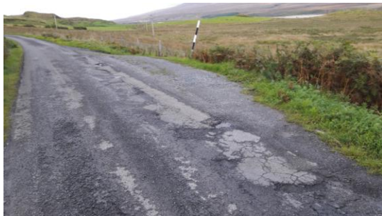
Resp3: an existing passing place on road to Bunnahabhain
